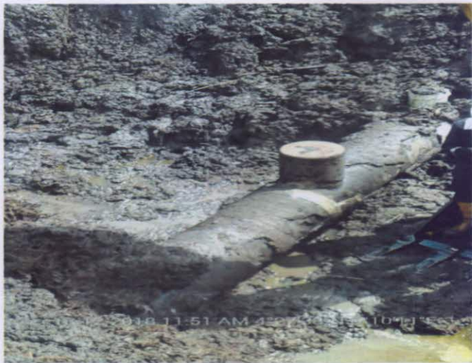
Figure 1: Replace Cone on the pipeline.
